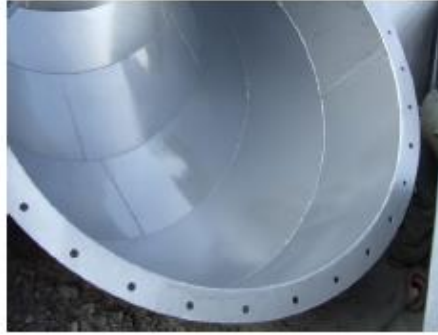
< RustGrip after 2nd coating>
