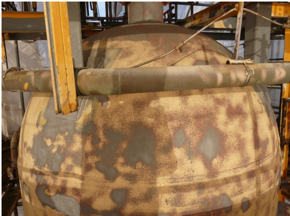
Sweep blasted surface before application
