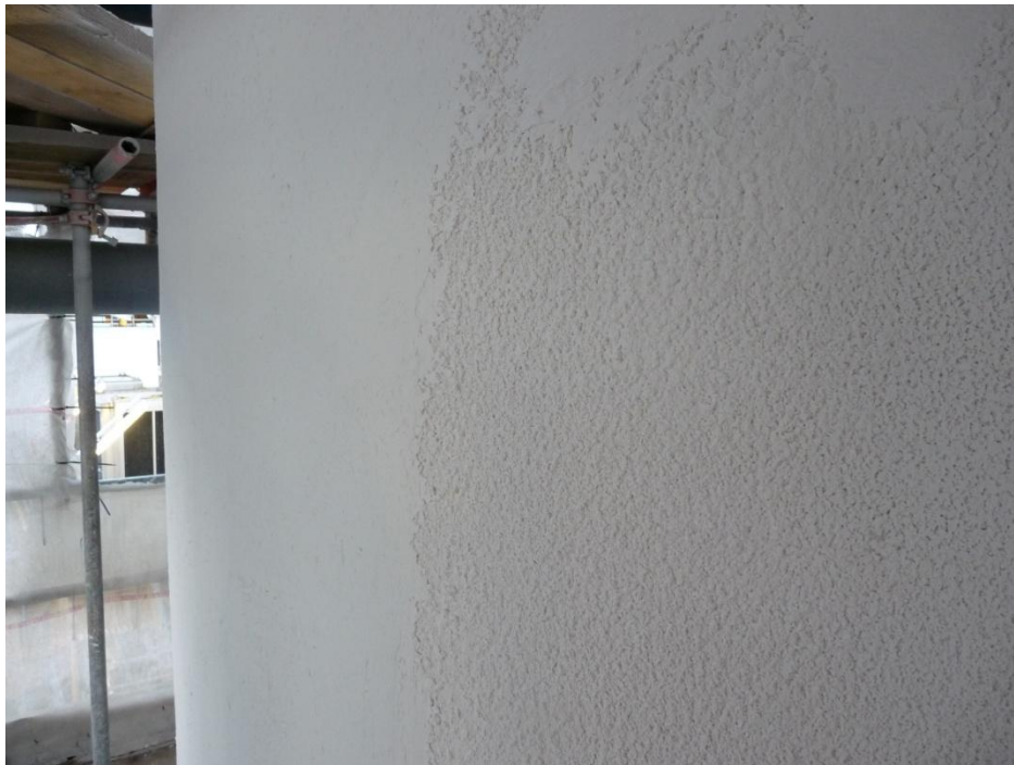
Surface partly troweled (left)
