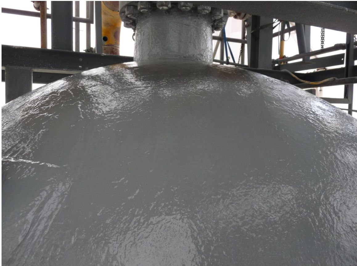
System completed with transparent coating TOP-E
