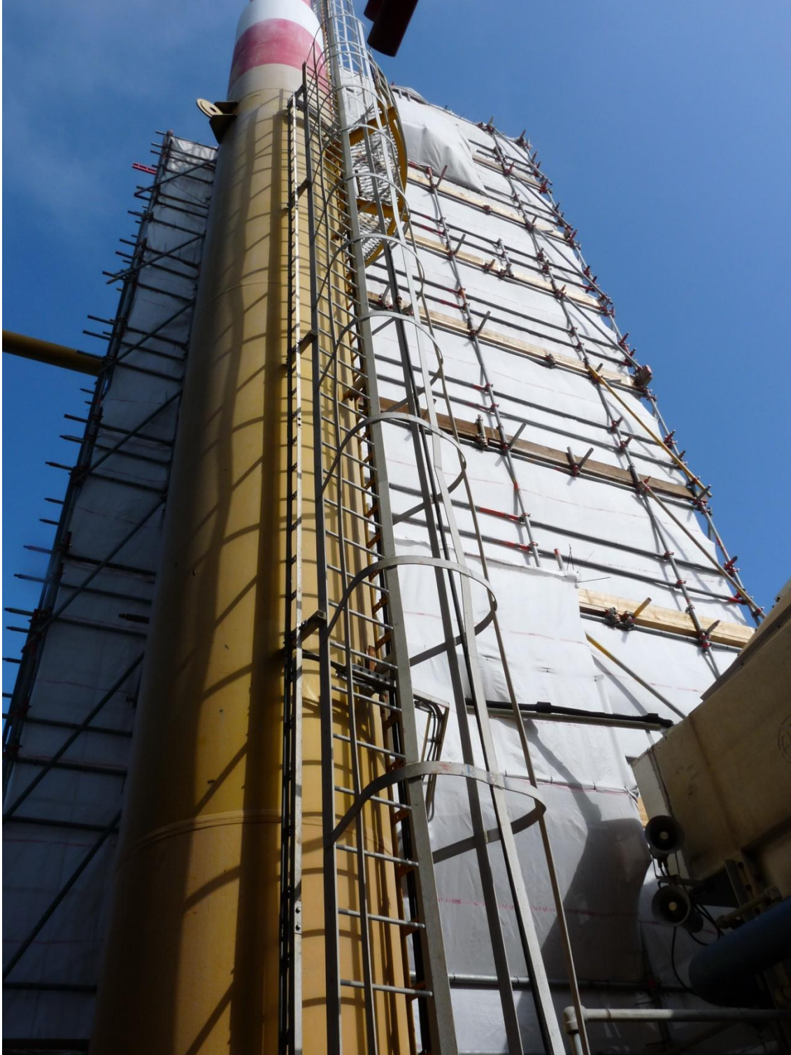
Vessel covered with scaffolding and tent
