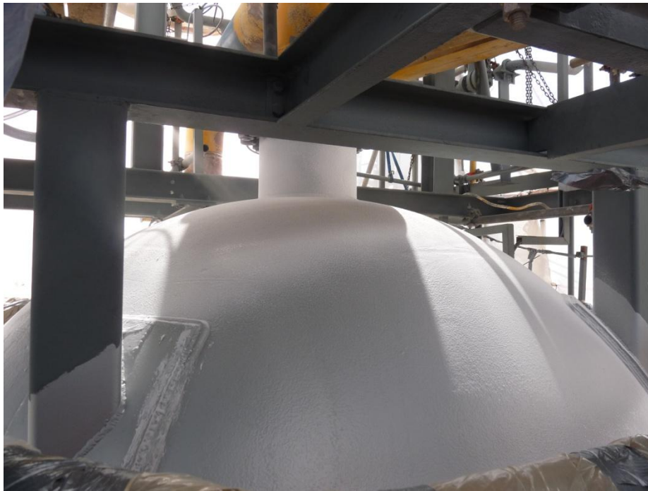
First layer of HSC at 1,5 mm
