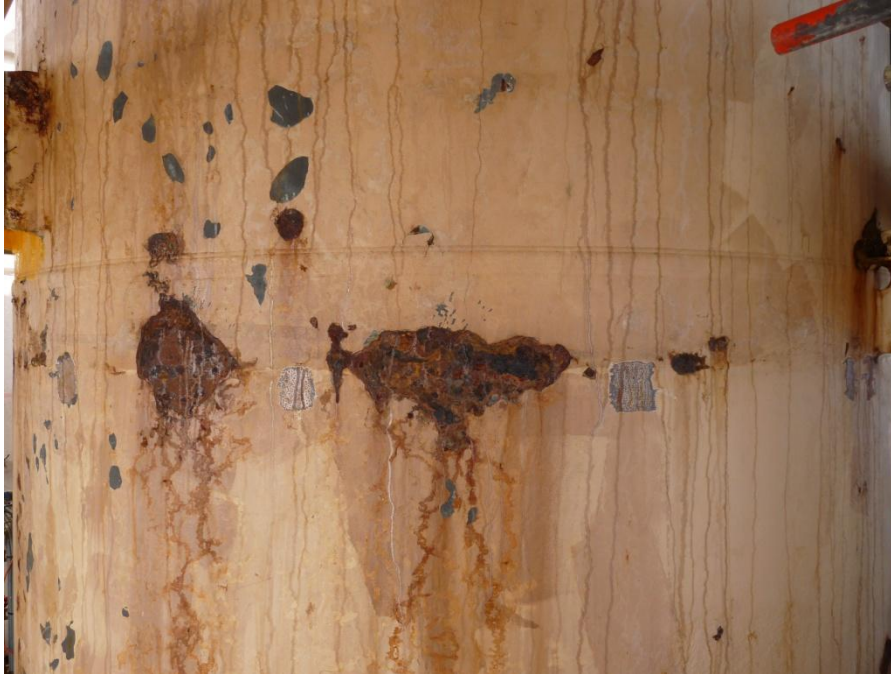
Corrosion under insulation (CUI)
