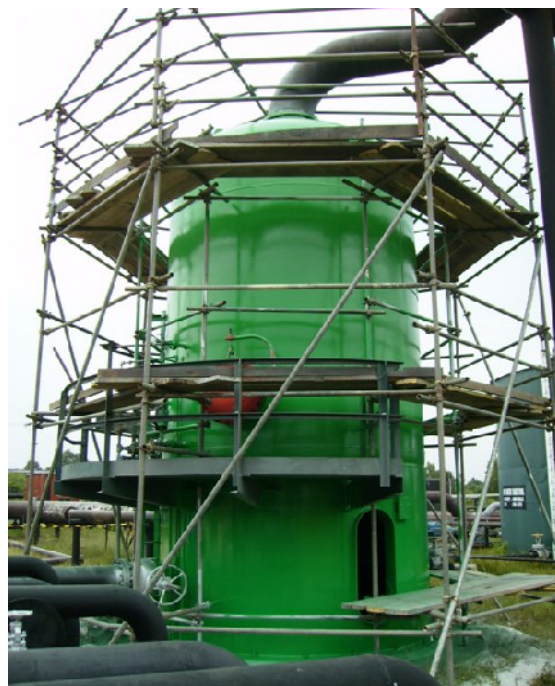
After applying RustGrip and EnamoGrip
