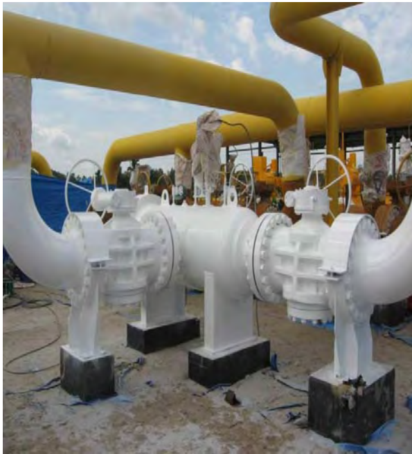
Application of Moist Metal Grip
