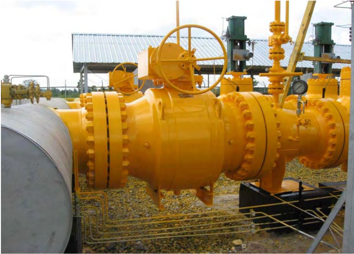
Application of Enamo Grip (safety yellow)
