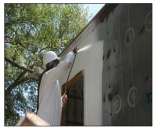
The exterior of the ISBU is sprayed with a ceramic coating that insulates the structure to reduce heating and cooling loads.
